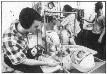
Before flight a Mercury astronaut's pressure suit was thoroughly tested.
