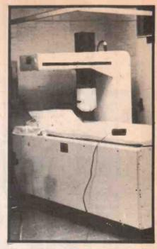
Fig. 10. This rectilinear scanner moves the single scintillation counter over the stationary patient: A typical scan could take up to half an hour.
