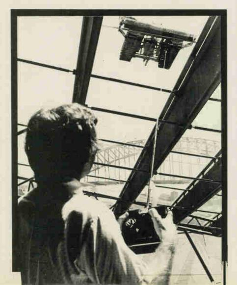
radio control of the vehicle was considered. An Australian company, Silvertone Electronics, were called in to provide a suitable radio control link, and assist in the electrical installation of all the control solenoids and switches.
