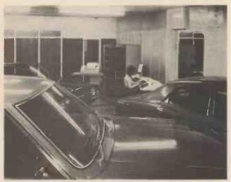
This computer, installed at a large car showroom in Glasgow, is used to correlate spare parts stocks with counter sales and workshop spares consumption. (Courtesy Digital Equipment Co. Limited.)
