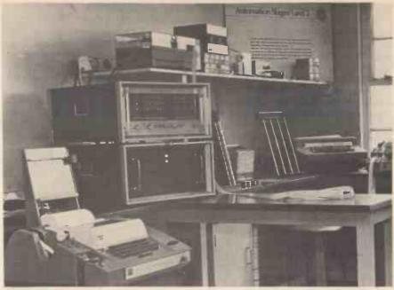
A Minic Computer in use at the laboratory of the Government Chemist. For analysis of the weight and moisture content of cigarettes and tobacco. This all-British computer was one of the first to use the "firmware" concept, in which the programming is simplified
