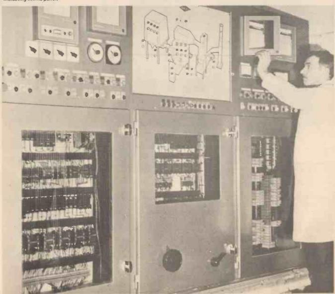
Fig. 9. Control console of Lucas automatic incinerator features indicating mimic panel.
