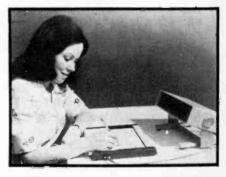
The Datapads are attached to miniprocessors which validate the data at source and indicate any errors to the user clerks via a screen. A 'clean' magnetic or paper tape is produced which is read directly into a main frame computer.
