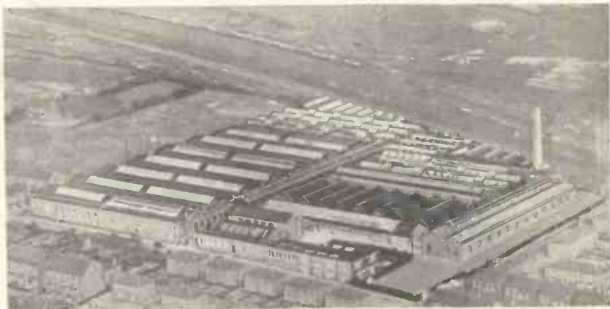
A built-up area of over 270,000 square feet is covered by the Moston, Manchester, factory of Ferranti, Ltd., which is entirely given over to the manufacture of radio.
