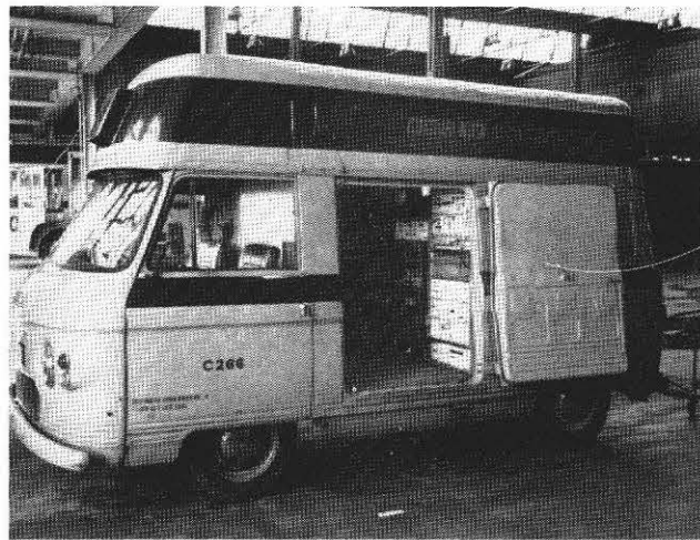
Fig. 1 Single-camera OB unit
