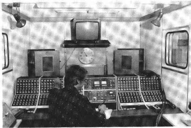
Fig. 3 General view of mixing console and monitoring equipment
