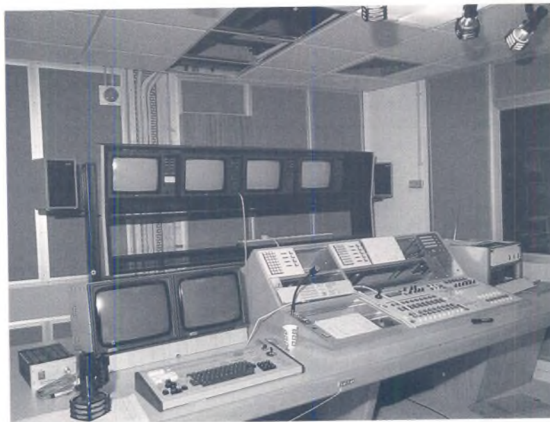
Continuity A nearing completion.
