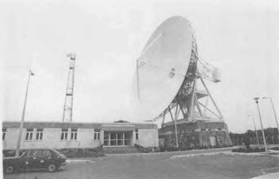
The Makarios ground station
