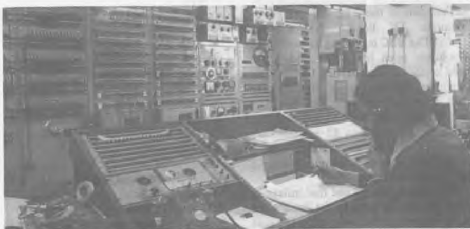
Julian Strickland, engineer, checking details of a reported fault, at the telecommunications fault position in the ATA
