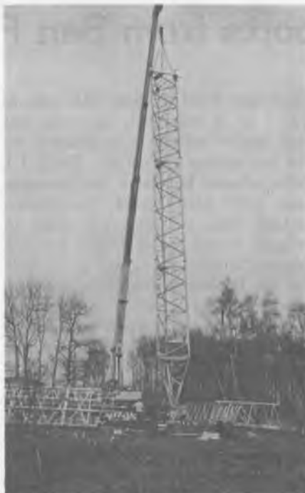
Re-engineering work at Wrotham continues. Here the new mast is being lowered onto a 4 inch steel ball bearing.
