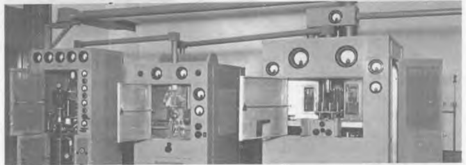
The Original Alexandra Palace transmitters
