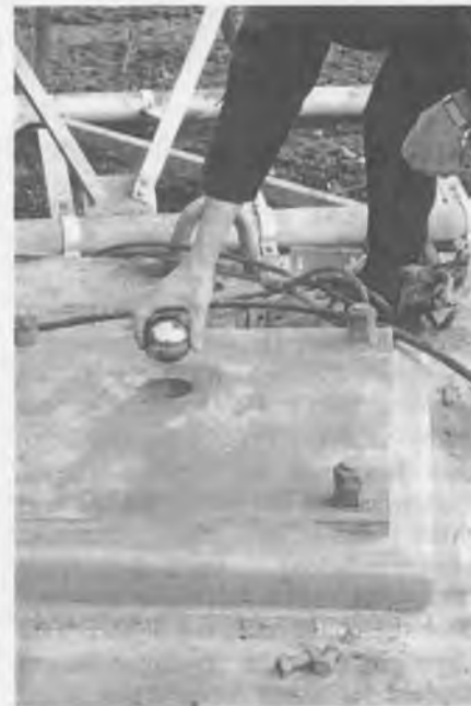
Re-engineering work at Wrotham continues. Here the new mast is being lowered onto a 4 inch steel ball bearing.
