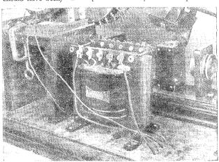
In a mains receiver it is necessary to arrange for the connections th a main received to the transformer to be tapped, so that the transformer can be adjusted to the voltage of supply—which may vary from 200 to 250 volts or more
