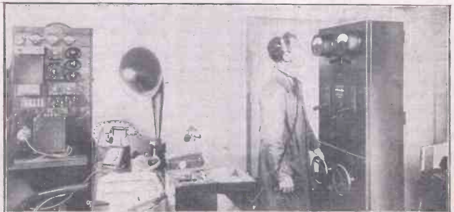
The Transmitting Room.
