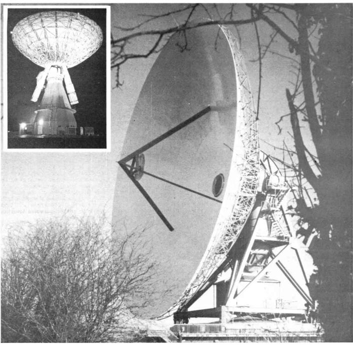
tion. This time made of aluminium, the dish measured 97 feet in diameter, and worked on the Cassegrain principle as did its predecessor. The unit moved in azimuth and elevation on bearings mounted at the top of a reinforced concrete tower six feet tall. The use of aluminium gave a further weight-reduction of the system to 331 tons.
