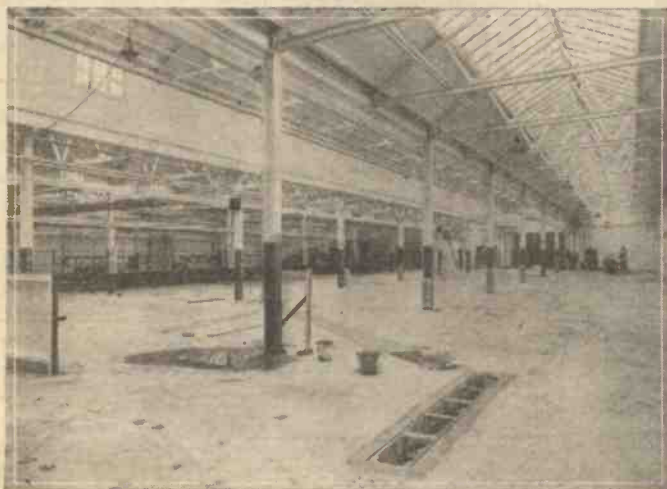
Part of the new Ferranti factory referred to on this page. This is the Valve Section.
