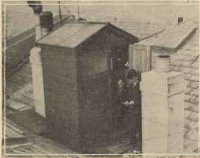
Picture of the special transmitting station erected on the roof of the Brighton police headquarters, from whence messages will be sent out and picked up by the policemen whilst on their beats. The pocket apparatus is now in operation at Brighton, which is the first town in the country to be equipped with the pocket radio.
