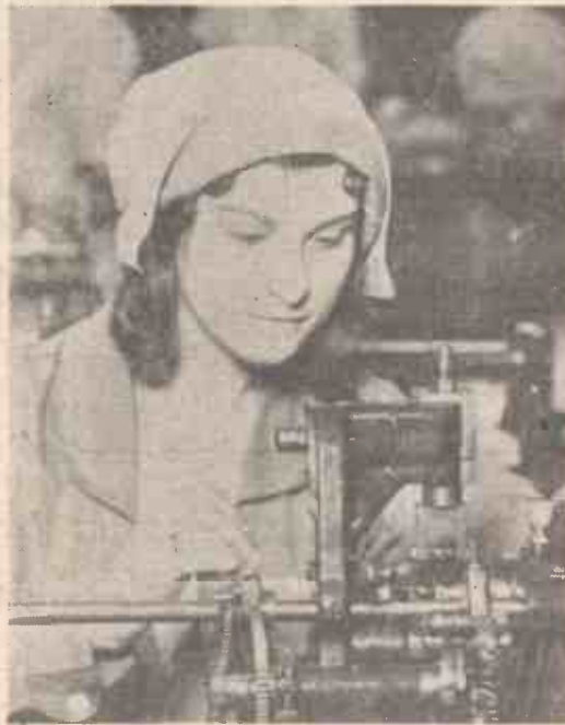
Fig. 3.—Winding the grid.
