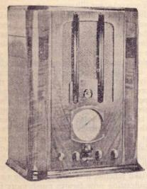
The Model T9-8 is identical to Model T9-7 except that the tuning range is from 155 to 320 kc/s., from 530/1,500 kc/s. and from 5,400 to 18,000 kc/s. There is also a slight modification in the tuned circuits to provide for the long-wave band.
