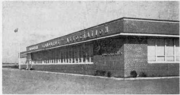
The CSA Testing Laboratory, Rexdale, Ontario. Building occupies over 60,000 sq. ft.
