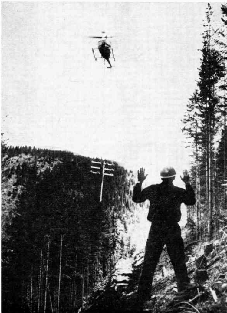
Figure 1. Crewman braces foot on stump to maintain balance as helicopter carries in pole for planting.
