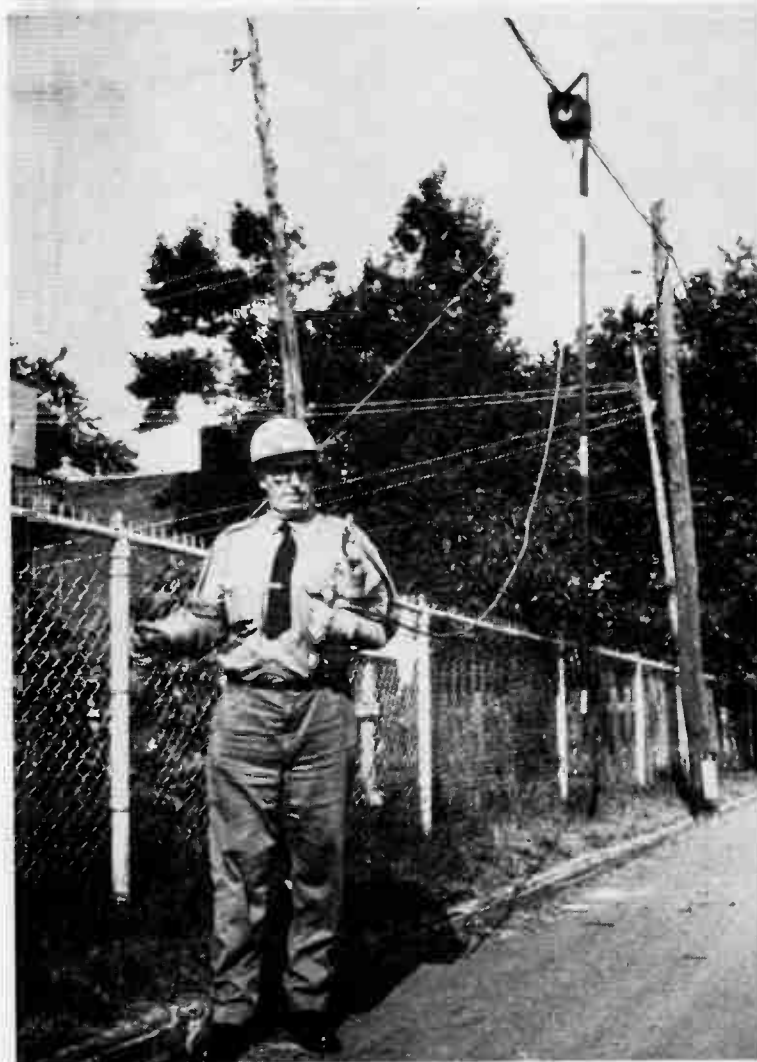
Figure 3. Gas collector moves along cable into which tracer gas has been injected. Operator watches flame for tell-tale indication.
