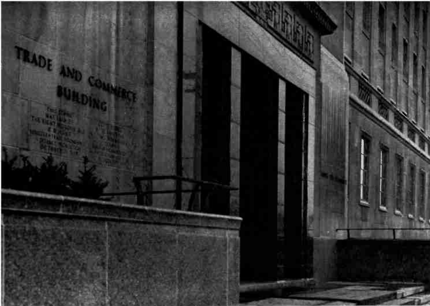
Headquarters building of the Canadian Department of Trade and Commerce in Ottawa. Officials of this department are expert in the knowledge of export techniques and are prepared to offer assistance to Canadian businessmen.
