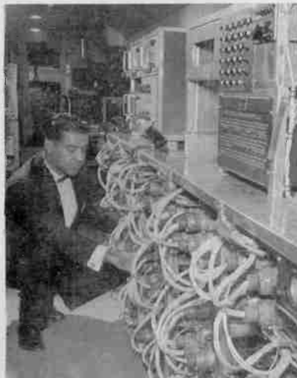
Two Convair T-29's have been modified for the specialized job of listening and talking aloft such as a missile would do. Convair's project engineer examines some of the miles of wiring connected with the electronic equipment which fills the cabin.
