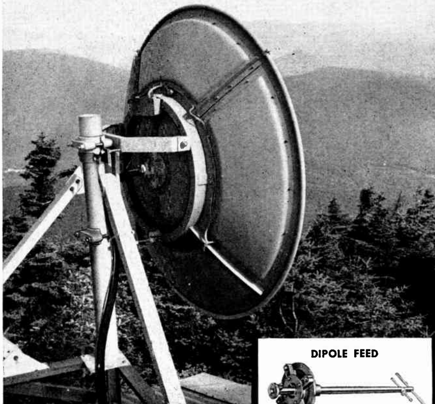
View of mountain top microwave installation
