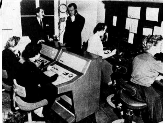
(Above) The cordless switchboard installed at Canadian Pacific Railway Company's London headquarters. The "key-sending" push-buttons can be seen next to the dial.
