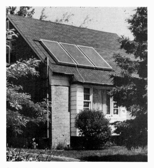
Four Ontario Housing Corporation houses are saving money through the use of roof mounted solar collectors which supply partially heated water to the existing water heaters. The systems cost under \$3000, in this case financed by the Ontario Ministry of Energy, who also supplied this photo.
