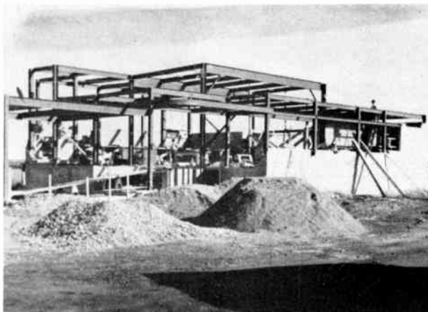
Lacombe was in steel framing stage in August, 1947.
