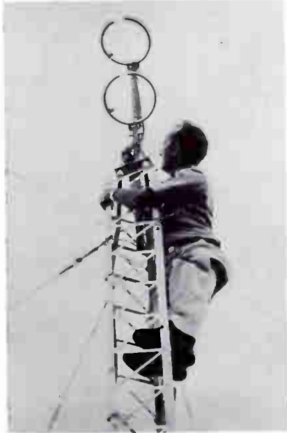
Fig. 2-15. Antenna Installation at United States Air Force TV Station, CSL-TV, Azores. The Rings are Separately Excited from Aural and Visual Transmitters. Official United States Air Force Photo.
