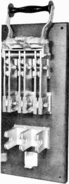
Fig. 5-19 shows a typical network sectionalizing switch, indoor type, rated at 7500 volts, 2000 amperes arranged with a latch and eye for hook-stick operation. This switch is commonly used for sectionalizing secondary networks of utility systems.
