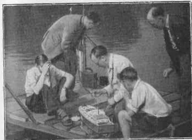
FIG. 78.—Model of an Admiral's barge being prepared to compete in an I.R.C.M.S. annual contest. This model employs a superhet circuit to enable simultaneous operation to be carried out with other models using this circuit.
