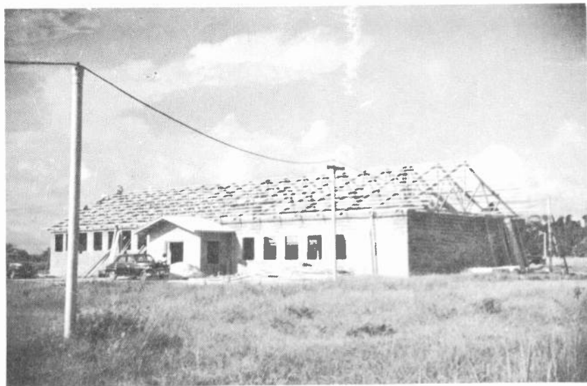
The building takes shape.
