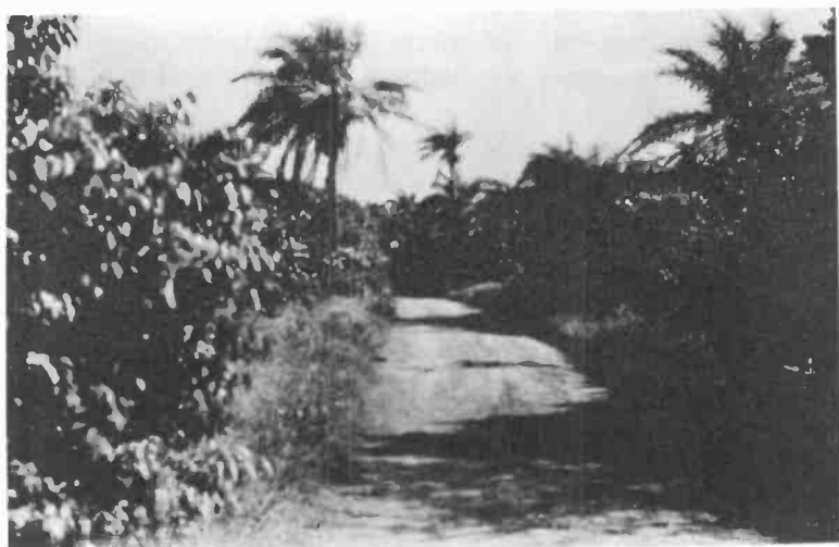
Our first road to ELWA's site — built by hand.
