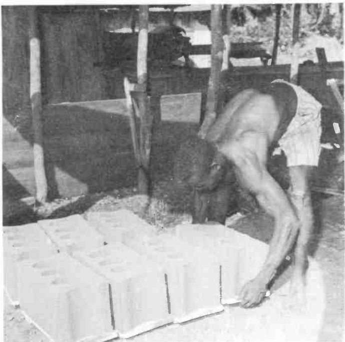
Thousands of cement blocks were made by a simple hand-operated machine.
