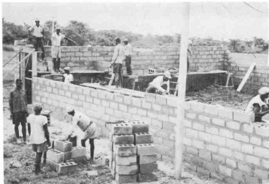
Construction gets underway.
