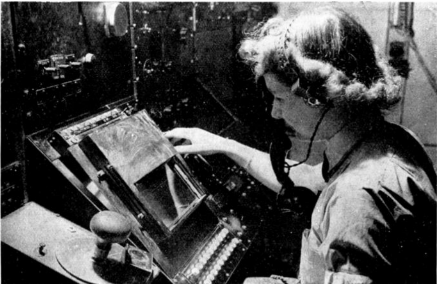
An airwoman plots a raider on a cathode-ray tube. Over 4,000 W.A.A.F. personnel were on radar duties during the war.
