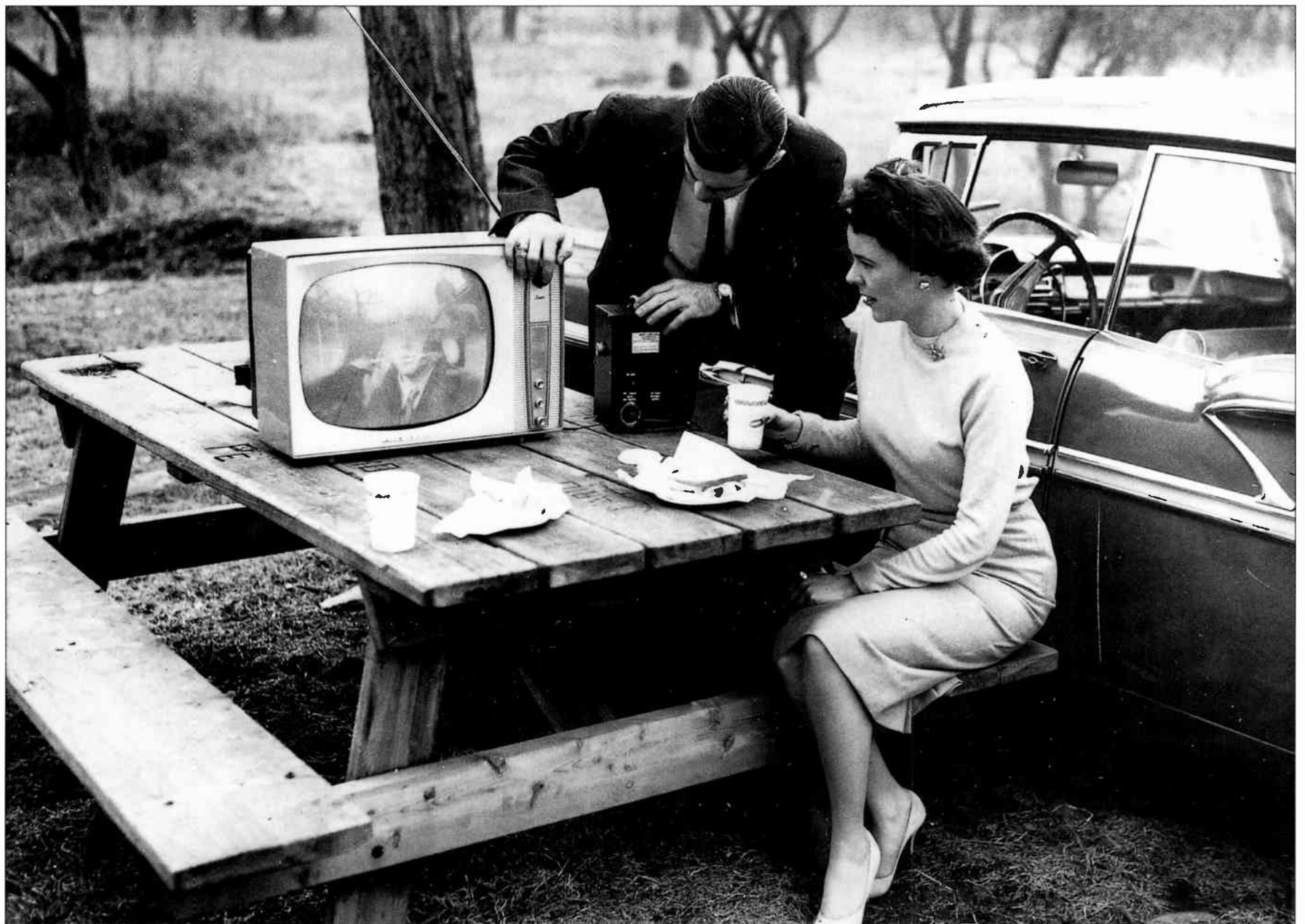
This portable TV set of 1954 plugged into a car's cigarette lighter socket.
