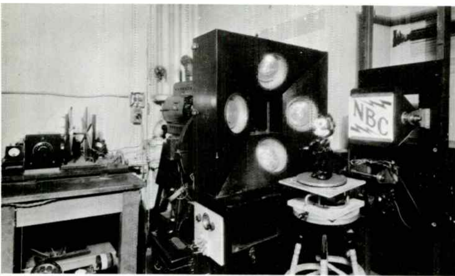
This 1930 photograph shows the entire operation—camera, personality (Felix the Cat on a phonograph turntable) and transmitter (on the table, to the left of the camera)—of W2XBS, which was the forerunner of NBC's New York outlet.
