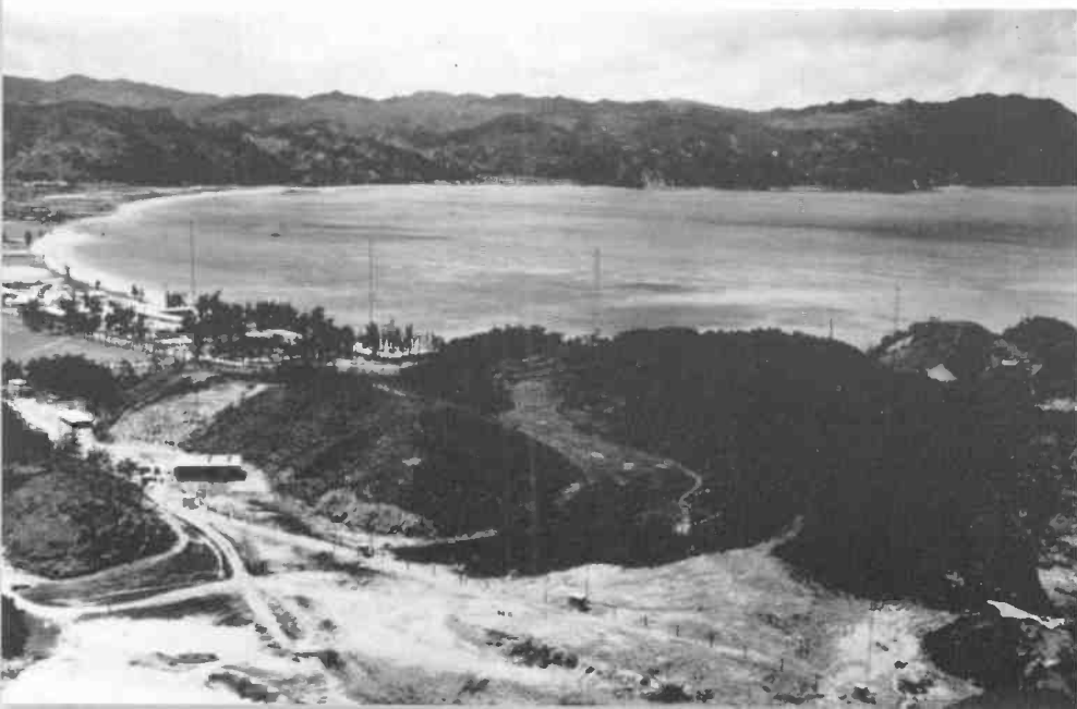
Aerial view of KSBU antenna area (four towers), Okuma, Okinawa.
