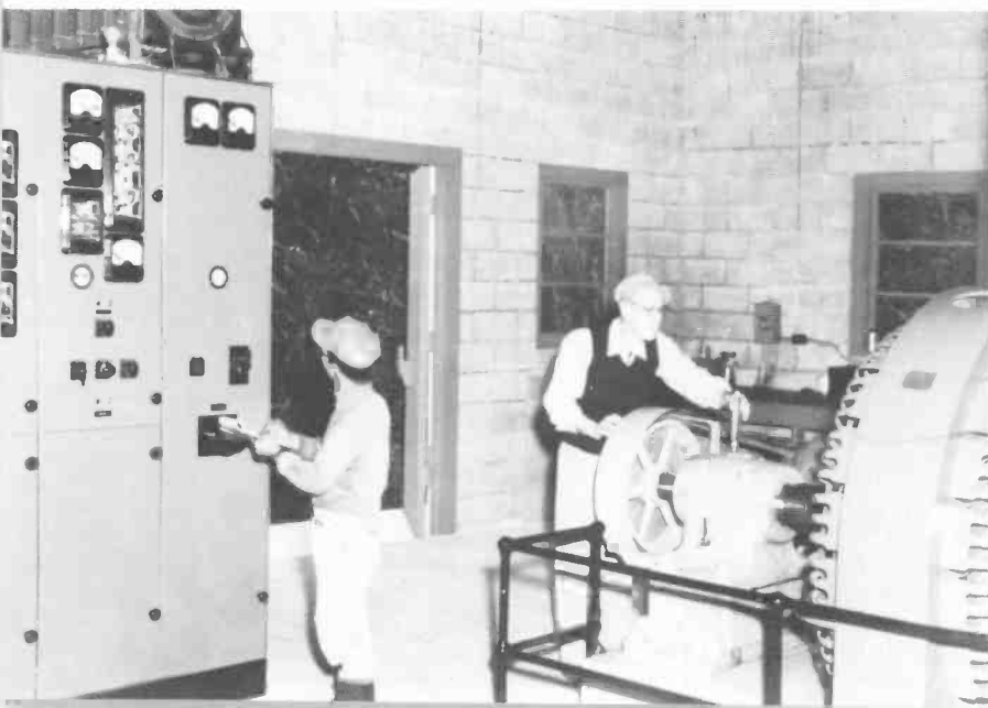
Diesel generator installed. Dick Caruthers, engineer, and his Ryukyuan assistant.
