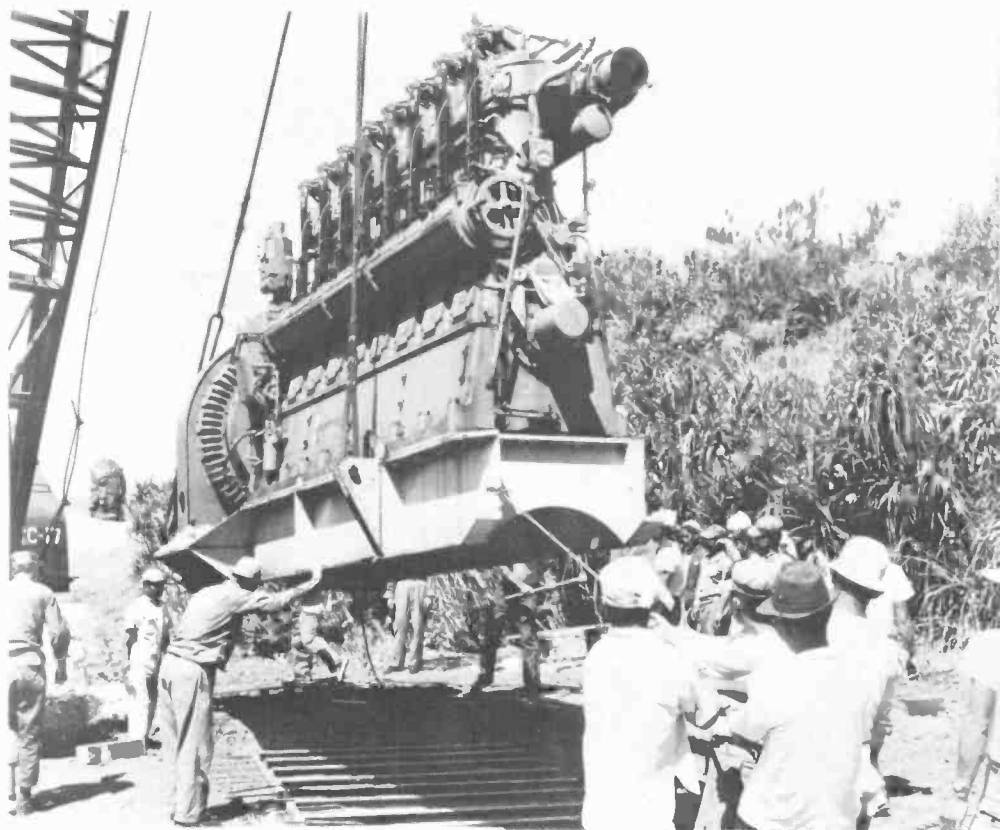
Installation of diesel generator over which building was later erected.
