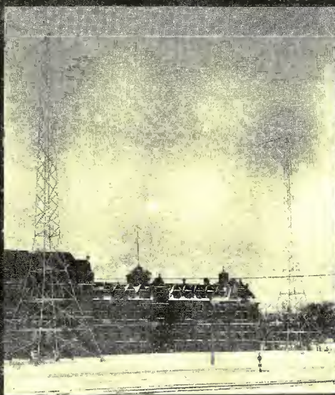
CANADIAN NATIONAL RAILWAYS BROADCASTING STATION AT MONCTON N.B.
