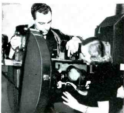
Mechanical scanning camera used by Dr. E. F. Alexanderson about 1930.
