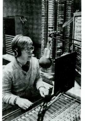
FIGURE 9.4 WHJJ/WHJY production studios. Although each studio is unique unto itself, the basics of layout are fairly consistent from station to station. For the sake of accessibility most studios are developed in a U shape, or a variation thereof.
