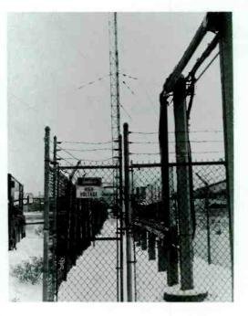
FIGURE 10.6 Lines leading from station transmitter to antenna base. FCC rules require fencing for safety purposes.
