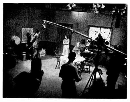
FIGURE 34. Scene from Colgate TV Theater. The use of the telescoping mike boom on which dialogue and sync sound are picked up considerably reduces the need for a soundman. (Courtesy of NBC-TV.)
