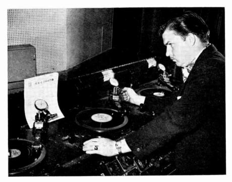
FIGURE 13. Fred Cole uses the "pre-set" indicator to find the exact groove on a sound record for an "inset" or "spot cue." (Courtesy of National Broadcasting Company.)
