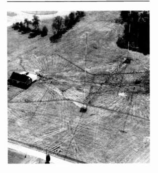
The entire steel tower of an AM radio antenna serves as its radiating element. For efficient propagation, its length must equal a quarter the length of the waves it radiates. Propagation also depends on soil conductivity, among other things. Heavy copper ground cables, buried in trenches radiating from the tower base, ensure good ground contact. The photo shows an array of antenna towers (for obtaining directional propagation) nearing completion, with the ground-cable trenching still visible.
