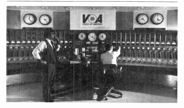
The master control panel, with its clocks showing the time in different world target areas, has long been the centerpiece of public tours of the Voice of America facilities at 330 Independence Avenue, S.W. in Washington, DC. A modern, solid-state, computerized facility replaced this old-fashioned, hands-on control panel in the 1980s, but it remains on show as part of the tour.
