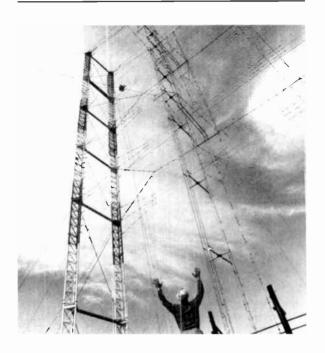
The Voice of America uses scores of short-wave antennas such as this. The steel towers support the cables that function as radiating elements. Each VOA site has many antennas to feed different frequencies in the HF hand, along with other suspended wires that act as reflectors to beam signals in specific directions to reach designated overseas target areas.
