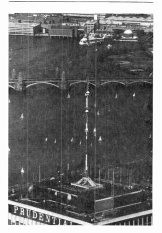
Because of the importance of beight to maximize television's line-of-sight coverage, Boston's WQTV (TV) chose the roof of the 55-story Prudential Center as its antenna site. A belicopter lifts the amenna assembly into place atop the supporting tower. The radiating elements are mounted in a spiral pattern, denoting circular polarization of the signal.
