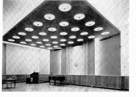
9. Dual AM-TV Studio,  $33' \times 45'$ , Two Stories High. It can be adapted for either radio or TV productions; walls include "splayed wing, as well as cylindrical reflectors. Resiliant, squeakless floor is made by 1' lengths of tongue-and-groove beech, fitted and held in place by mastic. An acoustical canopy is suspended above the work area. (Photo by courtesy of WGN, Chicago.)
