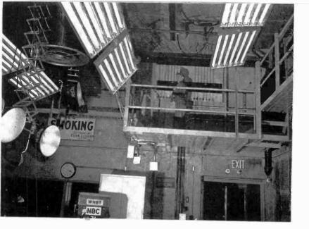
28. Lighting Crew at Control Switches. Lighting is controlled from central switchboard at WNBT. (Photo by courtesy of the National Broadcasting Company.)
