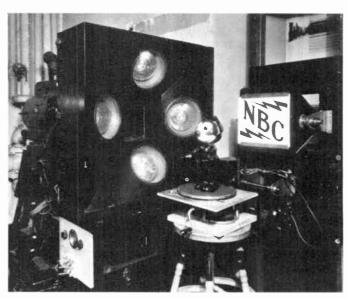
A 12-inch model of Felix the Cat (a popular cartoon movie character of the 1920s), posed on a revolving turntable, was used at the RCA laboratories as a moving subject to televise during the development of electronic television. The image at left shows how Felix looked on television in 1929 when picture definition was still only 60 lines per frame.
