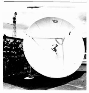
The most important technical development in the use of satellite distribution of video signals was the relatively small and inexpensive receive-only earth station, or TVRO. The dish collects and focuses the weak satellite signal for processing and boosting at the TV station, cable system, motel, or residence. Such dishes, thousands of which were in use in the early 1980s, are usually aimed at a single satellite (to cover two or more would add greatly to ground station costs).
