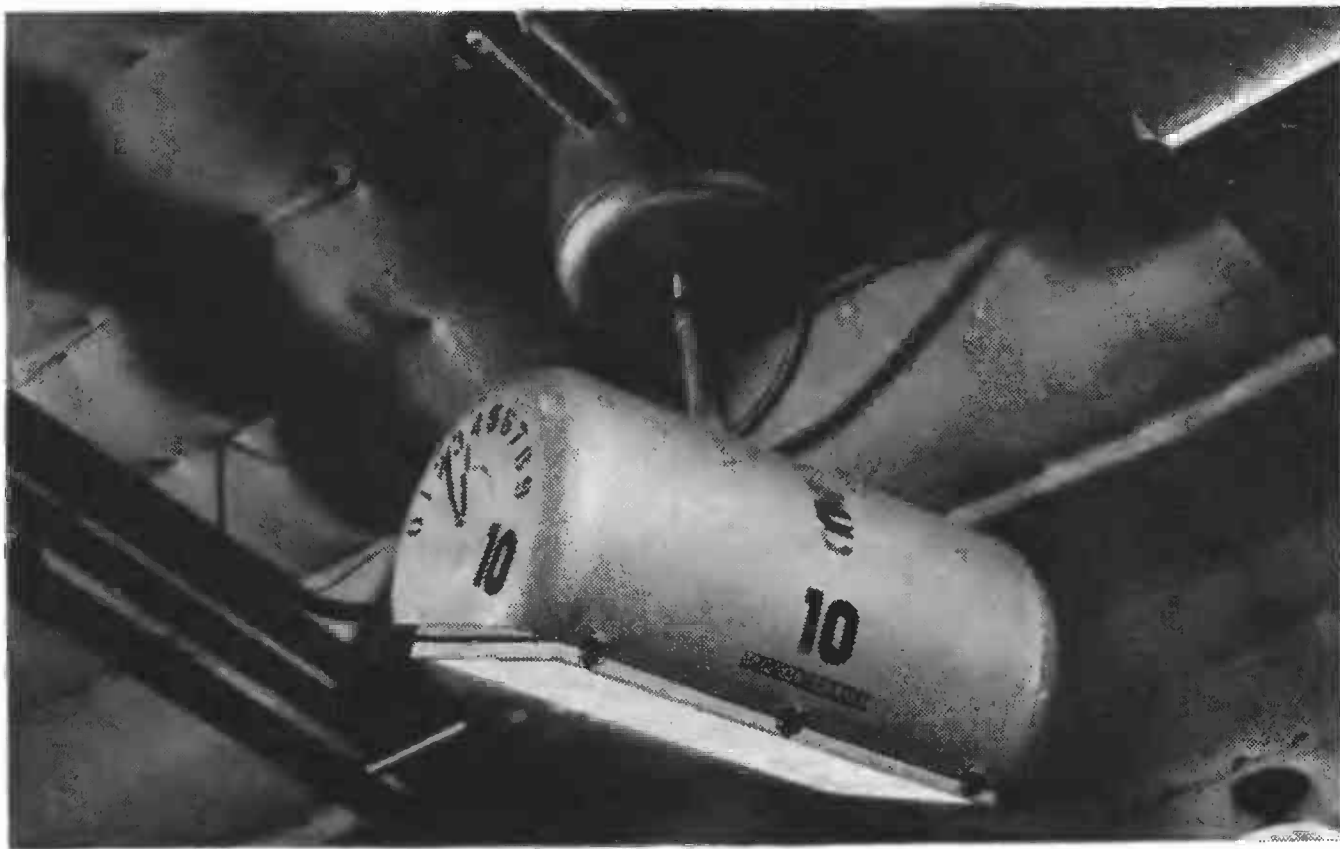
THE GENERAL ELECTRIC CEILING-MOUNTED HI-PRES-SURE MERCURY VAPOR LIGHT, MOTOR-CONTROLLED
