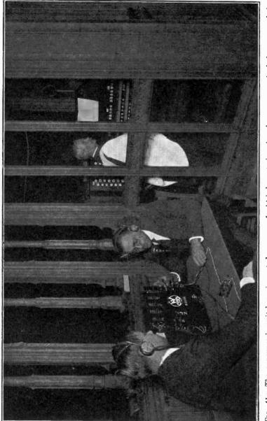
FIG. 41.—The announcer's switch equipment, by means of which he cuts in microphones, as required, for organ, choir, preacher and announcing, at a church service broadcast.
