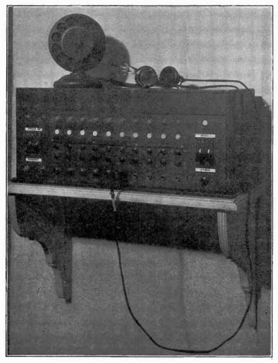
FIG. 35.—The studio switch equipment by means of which announcing for chain programs is controlled.
