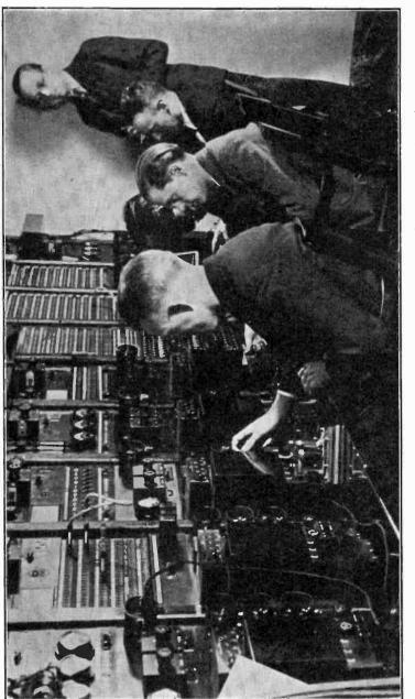
At the Fig. 33.—The input control equipment at WEAF, through which programs are supplied to stations all over the country. Ieft, five input amplifiers; at the right, the terminus of wire lines connected with distant broadcasting stations.
