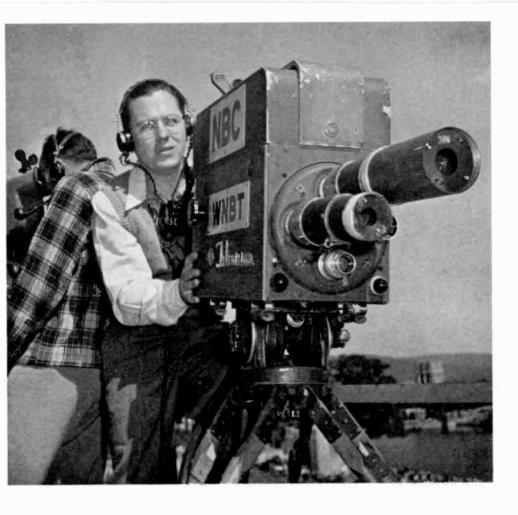
Typical television cameras in action during an outdoor telecast. The circular panel on which lenses are mounted is known as the turret. A simple mechanism throws the desired lens into action.
