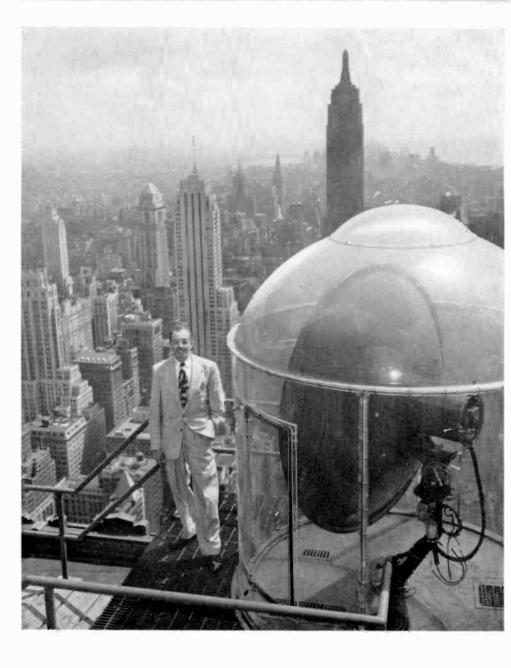
Chief Engineer O. B. Hanson, atop the RCA Building, inspects Radome, a parabolic antenna developed for micro wave relay between New York and distant cities.
