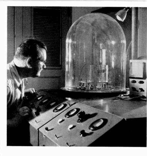
No other modern commercial industry leans so heavily on pure science as does television. Photo shows RCA scientist conducting an electronic research experiment on the evaporation of metals inside a vacuum chamber.
