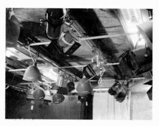
5.31 Pipe Grid: The pipe grid consists of rather heavy pipe strung either crosswise or parallel and mounted from 12 to 18 feet above the studio floor. The height of the grid is, of course, determined by the studio ceiling height, but even in rooms with low ceilings, the pipe should be mounted approximately two feet below the ceiling so that the lighting instruments or the hanging devices can be easily mounted onto the pipe.
