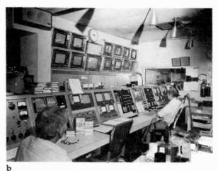
(except for live telecasts), and retrieves the appropriate program material for every second of the station's telecasting day. Additionally, master control is responsible for the technical quality of all program material being aired.
