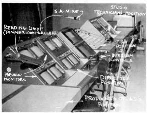
(master) and off-the-air monitors, intercommunication controls, audio monitor speaker controls, and an assortment of clocks and stopwatches.
