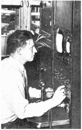
FIG. 49.—A monitoring position in the picture-bus truck. This is a piece of equipment similar to that described previously in connection with the live-talent studio equipment.
