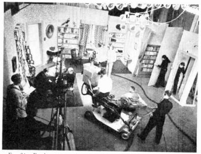
FIG. 84.—Further progress in "striking" Lestrade's office and making ready for next scenes. Notice Nathan's study is again complete. All of this scene shifting is done quietly while show is in progress.
