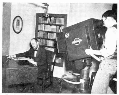
FIG. 29.—A book-review broadcast. While the commentator was turning pages, switches were made to close-ups of the various illustrations before another camera.
