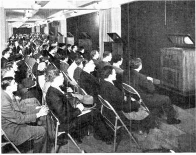
FIG. 28.—New York University students watching a televised lecture-demonstration on the principles of photoelectricity. The students, through a talkback circuit, were able to ask the lecturer questions just as in the classroom.
