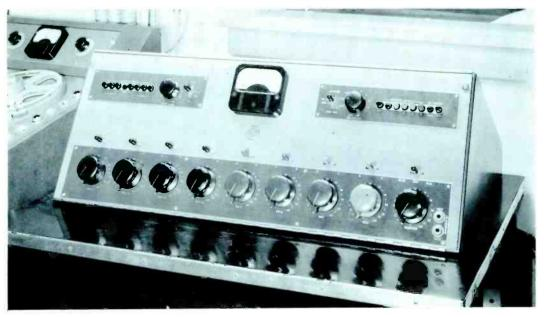
On the RCA Consolette, one of the most popular of the audio consoles, the monitor gain control is seen as a smaller dial on the upper left portion. The master gain control is in the extreme lower right. Pots number one through four, reading from left to right, are for microphones. Pots number five and six are for turntables number one and two. Pot number seven is for network input, and pot number eight is for remote lines.
