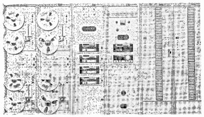
Gates automation system. A variety of programing formats can be handled through the combination of reel-to-reel transports, Criterion 80 cartridge decks, and the Criterion 55 multiple-cartridge reproducers.
