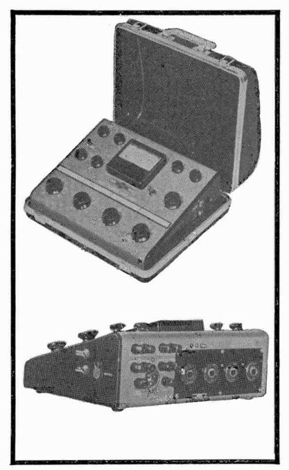
Collins four-channel remote amplifier powered by self-contained batteries with a life of approximately 75 hours. This unit is extremely portable.
