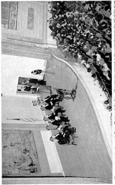
The stage is set for America's Town Meeting of the Air. Of particular interest is the microphone on the left of the stage equipped with the parabolic reflector. This is pointed toward speakers in the audience to piok up their voices and deflect them directly into the microphone.
