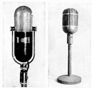
Left.—Uni-directional microphone (RCA Type 77-B). (Courtesy of RCA.) Right.—Western Electric's new "cardioid" uni-directional microphone, (639-A) combines in one instrument the pickup characteristics of a monodirectional, bi-directional and a non-directional microphone. Either of the effects may be selected by operating a small rotary switch set flush in the surface of the housing. (Courtesy of Western Electric Company.)
