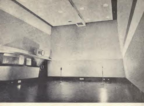
Figure 7. Live-end dead-end studio with slanting walls.
