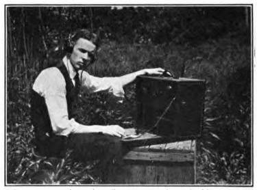
Government market and weather reports can be received by an amateur radioist out in the open field, using an aerial made by tossing a wire over the limb of a tree.
