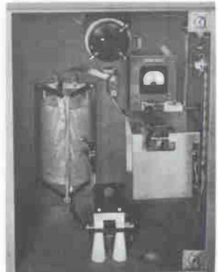
Fig. 7-5. A typical antenna tuning unit. The lighting choke is at the top of the cabinet.
