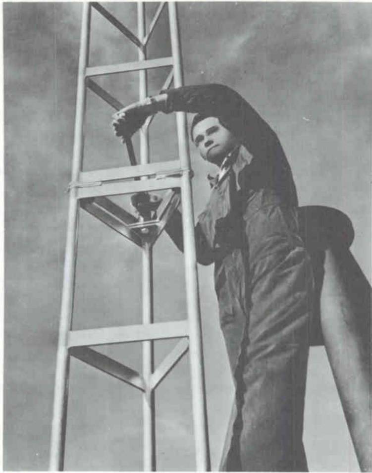
Fig. 5-8. Tower sections must be tightly bolted together to provide good electrical conductivity.
