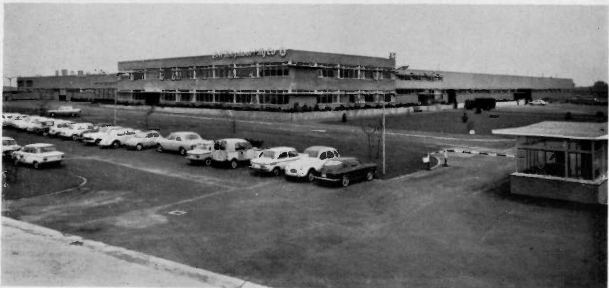
Figure 4—New Frigibell refrigerator factory at Geel in Belgium.
